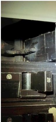
Electrical: Disintegrated electrical bar.
