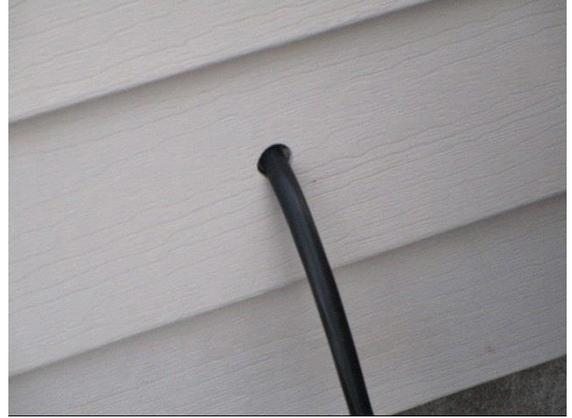
Exterior Surface: Unsealed entry into siding.
